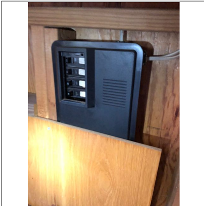
Small sub panel located in shed.
