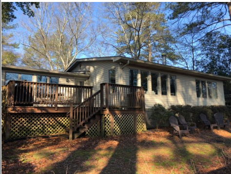
Rear elevation of house.
