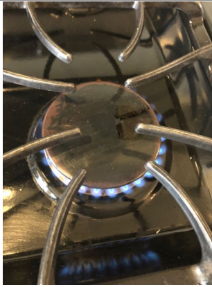
The right front burner on the stove has poor gas flow. Recommend repair by qualified appliance repair technician.
