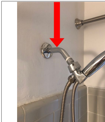
The shower spout was loose. Recommend repair by qualified plumber.
