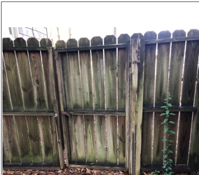
The gate on the left elevation of the house was not operable. Recommend repair by qualified carpenter.
