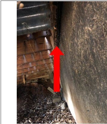
Unable to determine deck attachment to House. Recommend evaluation and repair by qualified contractor.
