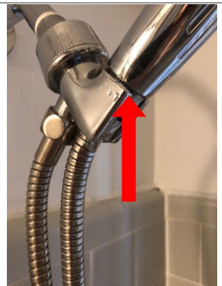
Recommend tightening the shower head.
