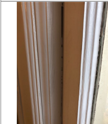
The window was painted shut.
