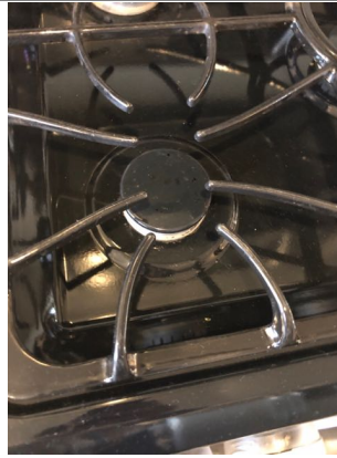
The striker for the left front burner on the stove does not work properly. Recommend repair by qualified appliance repair technician.
