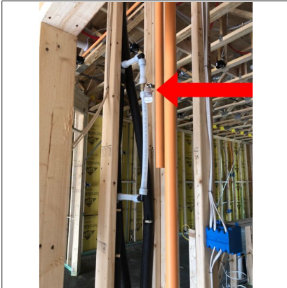
Water main shut off and sprinkler system located in garage closet.
