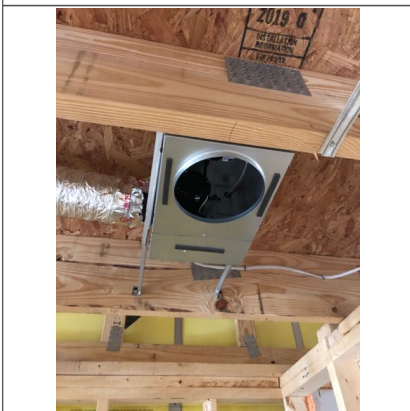
Rough exhaust fan.
