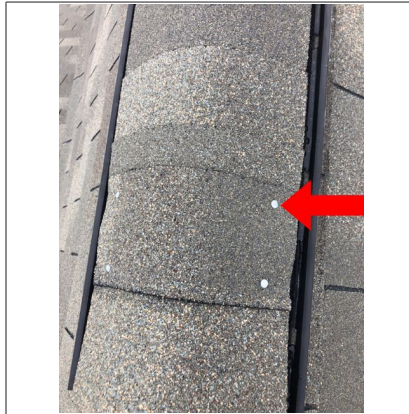
Recommend sealing the exposed nail heads on the ridge shingles.
