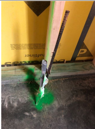
Rebar on the left wall that according to the builder will be removed.
