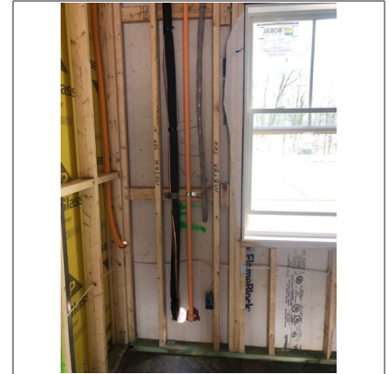
Electrical entry on back wall.
