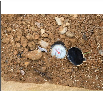
Water meter located at street
