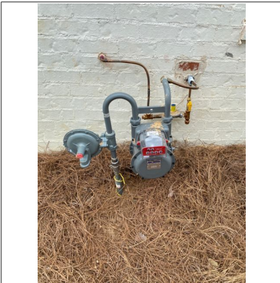
Main fuel shut off and gas meter located on right side of house
