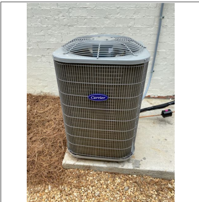
Exterior AC unit two was front unit located on right side of house
