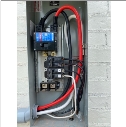
Interior of main electrical panel two located on right side of house
