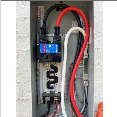
Interior of main electrical panel one located on right side of house
