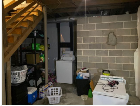
Rear foundation wall 4928
