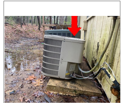
The exterior AC unit for 4926 was not level. Recommend repair by qualified HVAC technician.
