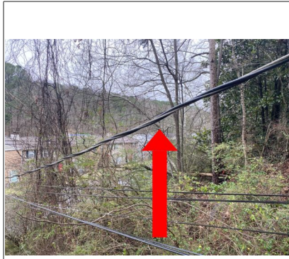
The main electrical service cable could be reached from the porch of 4926. Recommend repair by qualified electrician.
