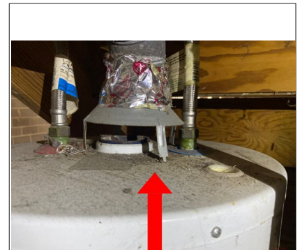
The draft hood on the water heater for 4926 was not mechanically fastened to the top of the water heater. Recommend repair by qualified plumber.
