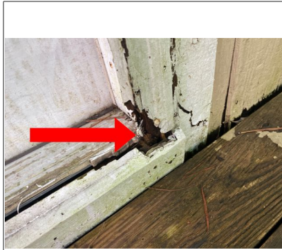
There was moisture damage on the siding and trim in many areas on the rear side of the building. Recommend repair by qualified carpenter.
