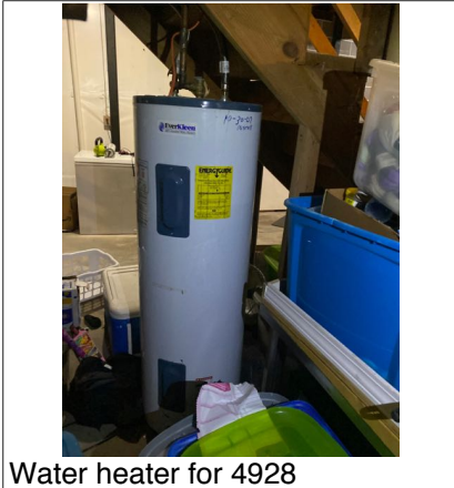
Water heater for 4928
