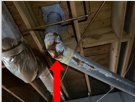
There was corrosion on the vent pipe for the furnace for 4926. Recommend repair by qualified HVAC technician.
