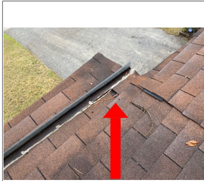
There was moisture damage on the left side of the porch roof for 4928 and the shingle was damaged. Recommend repair by qualified roofer.
