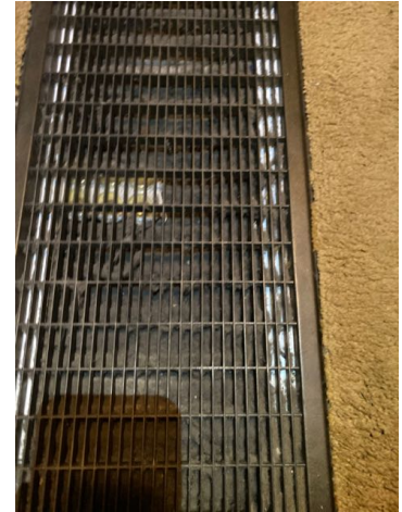
Recommend replacing the air filters
