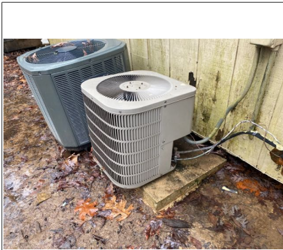
Exterior AC unit for 4926 located on rear side of building
