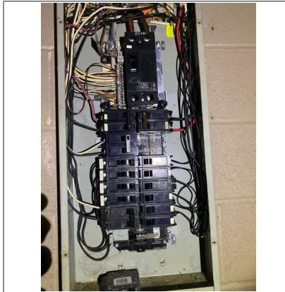
Interior of electrical panel for 4928 located in basement
