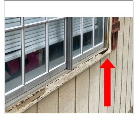
There was moisture damage on the soffit and window trim on the front side of the house. Recommend repair by qualified carpenter.
