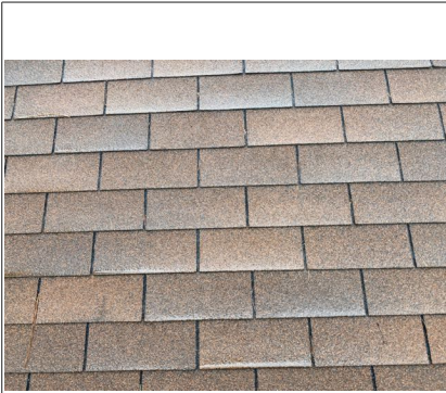
Overview of shingle condition
