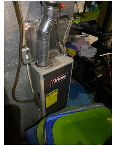
Interior HVAC system for 4928 located in basement
