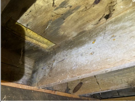
There was possible fungal growth on the framing in front of the porch in 4926. Recommend evaluation/repair by mold remediation specialist.
