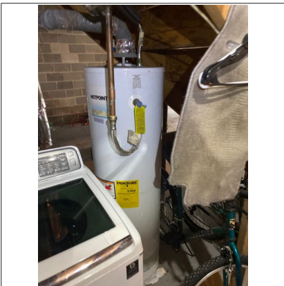
Water heater for 4926
