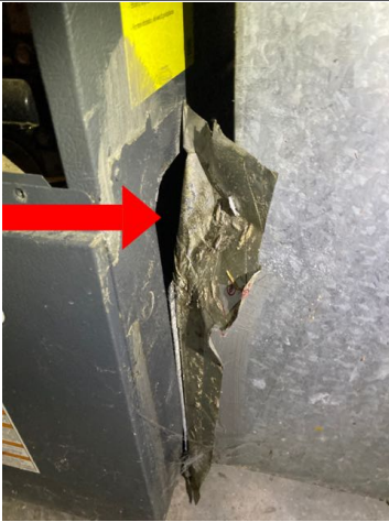
The return ductwork at the furnace for 4926 needed to be re-taped. Recommend repair by qualified HVAC technician.
