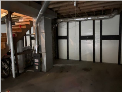
Rear foundation wall 4926
