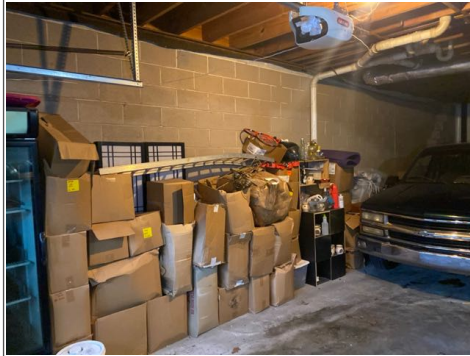
Left foundation wall 4928
