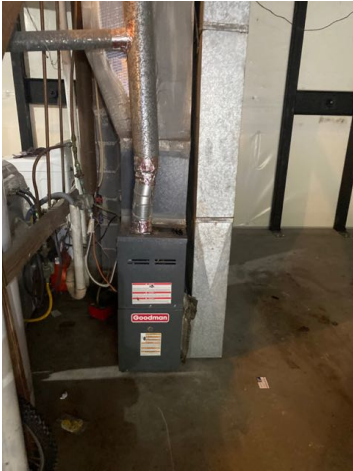
Interior HVAC system for 4926
