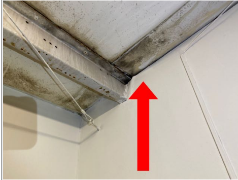
There was moisture damage on the bottom of the front wall in the upper right room from an active roof leak. Recommend repair by qualified contractor.
