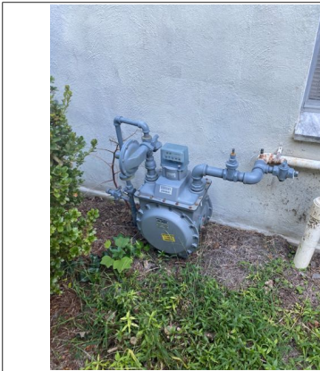
Main fuel shut off and gas meter located on front side of building
