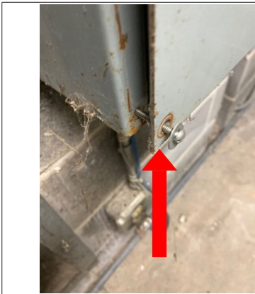
Recommend installing appropriately sized fasteners on the dead front cover for electrical sub panel one.
