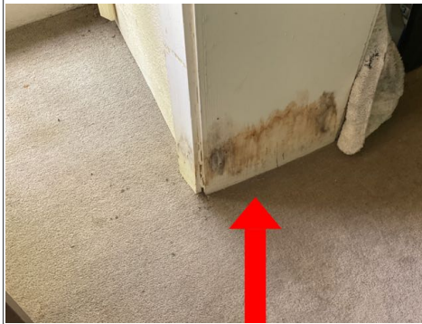
There was old moisture damage on the bottom of the trim on the left side of the Police Department closet.
