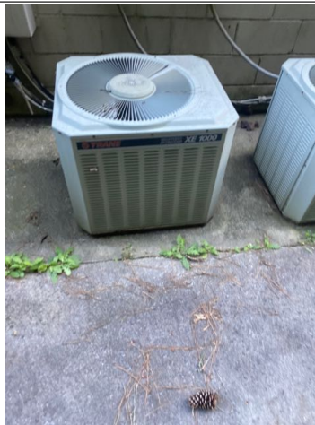
Exterior AC unit seven located on right side of building
