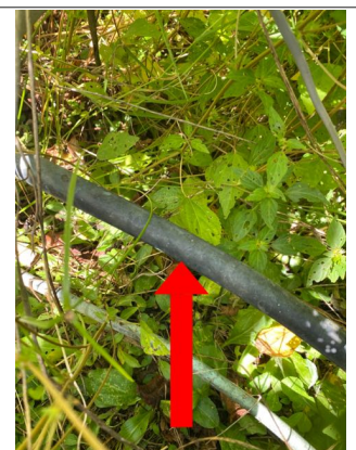
Recommend replacing the insulation on the suction line for exterior AC unit four.
