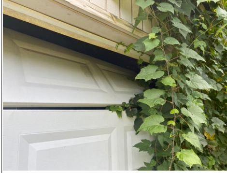
The rear left garage was in overall poor condition.
