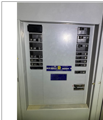
Interior of electrical sub panel two located in right side of building
