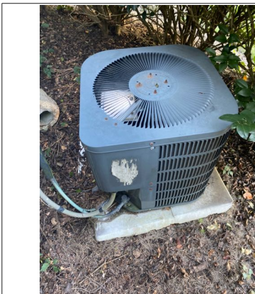
Exterior AC unit one located on left side of building
