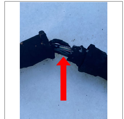
The conduit protecting the electrical wires to exterior AC unit four was damaged. Recommend repair by qualified electrician.
