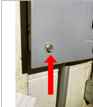
Recommend installing properly sized fasteners to secure the dead front cover to electrical panel one.
