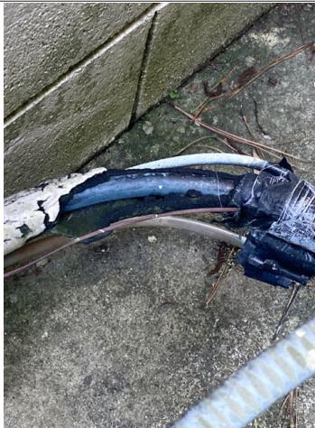
Recommend replacing the insulation on the suction lines on all of the exterior AC units.
