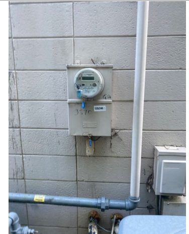
Main electrical service entrance located on right front side of building
