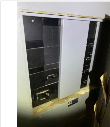
Main electrical disconnects located in right side of building
