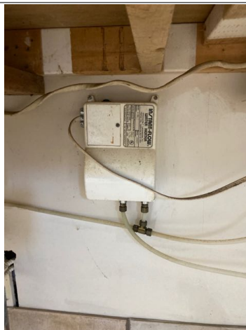
The water heater for the sinks in the women's bathroom did not appear to be working. Recommend repair by qualified plumber.
