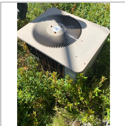
Exterior AC unit four located on left side of building
