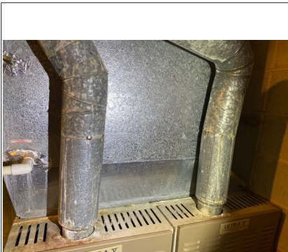
Unable to determine the age of interior AC unit five because the manufacturer's data plate was not visible.
