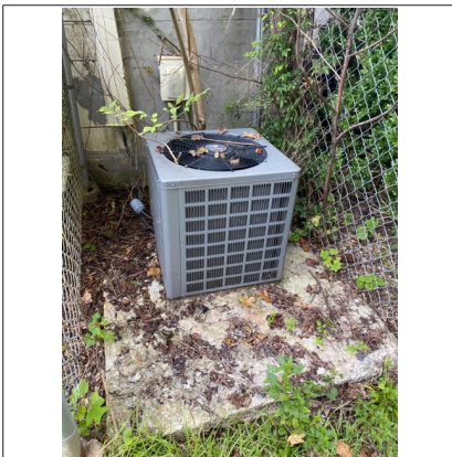
Exterior AC unit one located on right side of building
