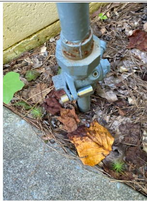
The gas meter was locked.
