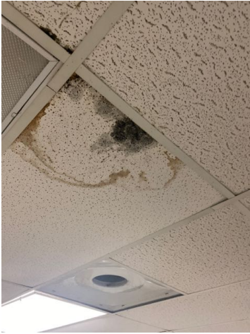
There was possible fungal growth on the ceiling throughout the building. Recommend evaluation/repair by mold remediation specialist.
