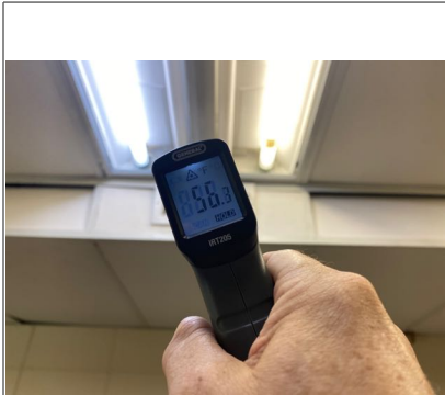
Air conditioning system four temperature at register
