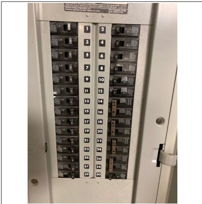
Electrical sub panel four located in rear side of building
