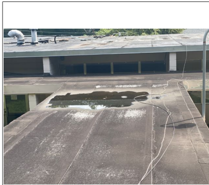
Water was ponding on the rear left side of the walkway covering the rear side of the courtyard. Recommend repair by qualified roofer.
