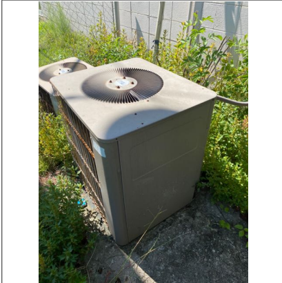
Exterior AC unit three located on left side of building
