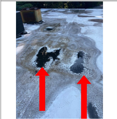
Water was ponding in several areas on the flat roof. Recommend evaluation/repair by qualified roofer.
