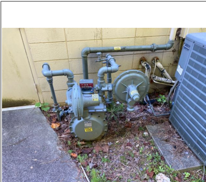
Main fuel shut off and gas meter located on right side of building
