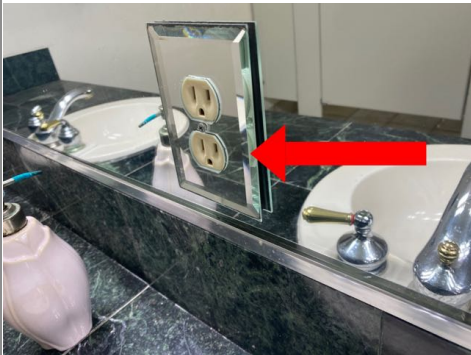
The electrical receptacles in the women's restroom were loose. Recommend repair by qualified electrician.
