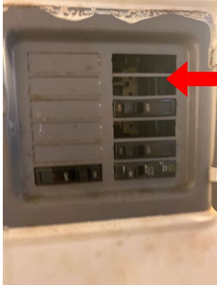
Several breaker filler plates were missing in electrical sub panel two. Recommend repair by qualified electrician.
