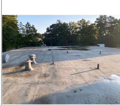
Front roof overview
