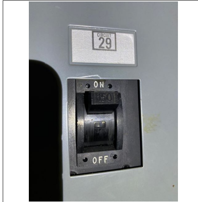
Main electrical disconnect one
