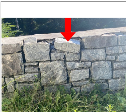
Several of the stones in the retaining walls on the right side of the building were loose. Recommend repair by qualified brick mason.
