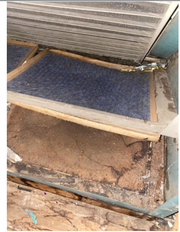
Recommend replacing the air filters.
