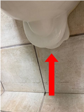
The drain for the right urinal in the men's restroom was leaking. Recommend repair by qualified plumber.
