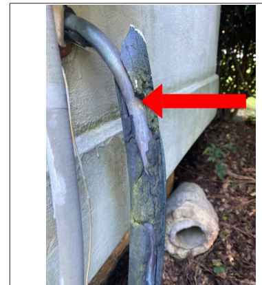
Recommend replacing the insulation on the suction lines for all of the exterior AC units.
