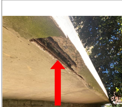
The concrete below the gable on the rear left side of the building was damaged. Recommend repair by qualified brick mason.
