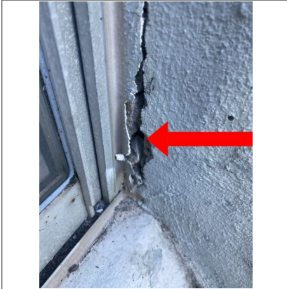
Recommend sealing the opening on the lower right side of the window next to the left entry door.
