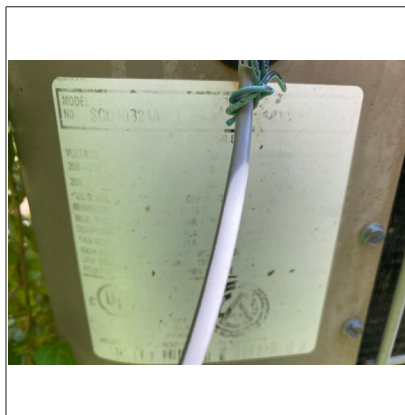
Unable to determine the exact age of exterior AC unit four because the manufacturer's data plate was not legible. It appeared to be 20+ years old.
