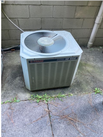
Exterior AC unit eight located on right side of building
