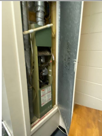
Interior HVAC system four located in rear left side of building
