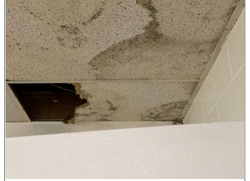
There was possible fungal growth on the ceiling in the rear left room. Recommend evaluation/repair by mold remediation specialist.
