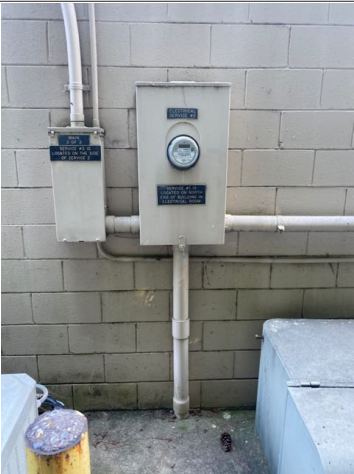
Secondary electrical service entrance located on right rear side of building
