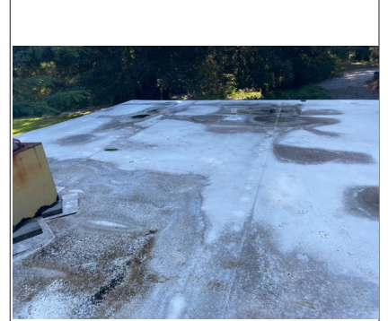
Overview of flat roof
