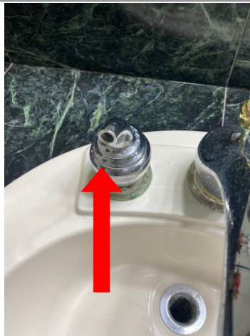
The hot water handle on the left sink in the women's bathroom was missing. Recommend repair by qualified plumber.
