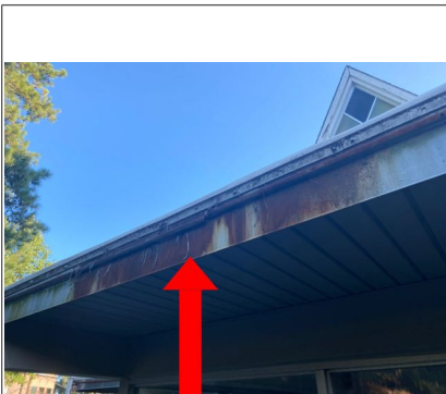
There was corrosion on the lower fascia on the front side of the building. Recommend painting.
