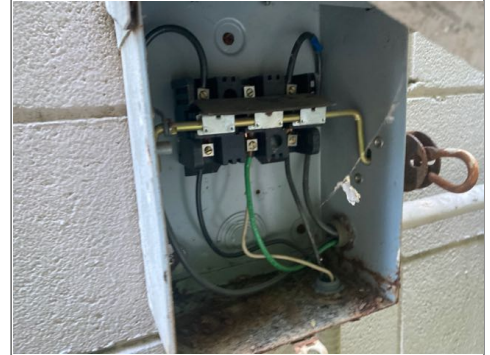
Dead front covers were not mechanically fastened to all of the electrical disconnect boxes for the exterior AC units. Recommend repair by qualified electrician.
