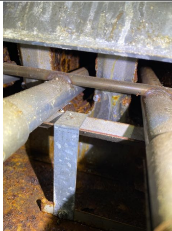
There was heavy corrosion inside furnace two. Recommend evaluation/repair by qualified HVAC technician.
