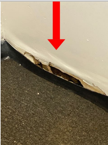
There was moisture damage on the bottom of the front wall in the upper right room from an active roof leak. Recommend repair by qualified contractor.
