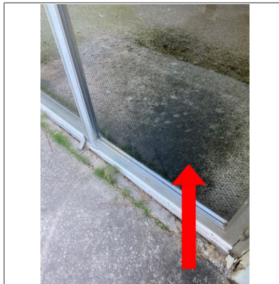
The grading was negative on the front side of the building and surface water appear to be entering through the entry doors. Recommend repair by qualified contractor.
