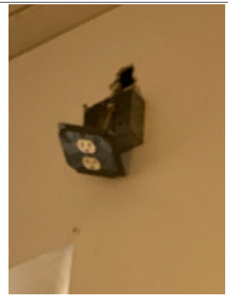
The upper electrical receptacle on the rear wall of the sanctuary was not securely attached. Recommend repair by qualified electrician.
