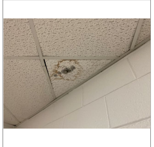
There was active moisture damage on the ceilings throughout the building. Recommend repair by qualified contractor after the roof is repaired.
