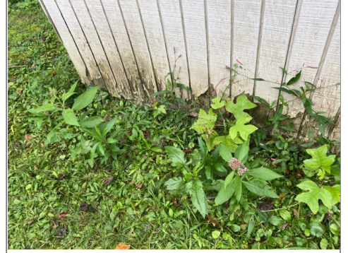
The rear left garage was in overall poor condition.
