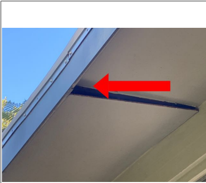
The soffit was loose in several areas on the right side of the building. Recommend repair by qualified carpenter.
