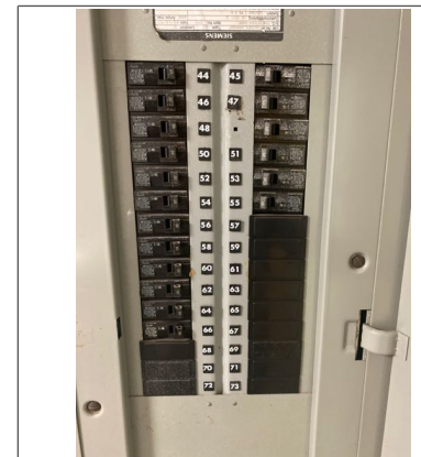
Electrical subpanel three located in rear side of building
