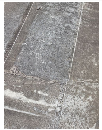
Most of the rolled roofing on the walkway covering was in poor condition due to cracking. Recommend evaluation/repair by qualified roofer.
