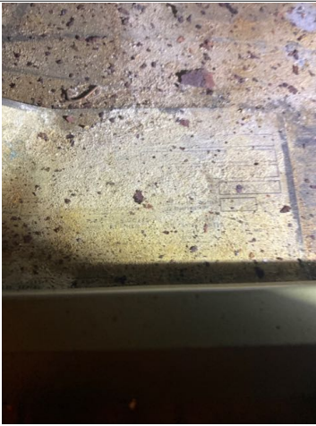
Unable to determine the exact age of furnace four because the manufacturer's data plate was not legible. It appeared to be 40+ years old.
