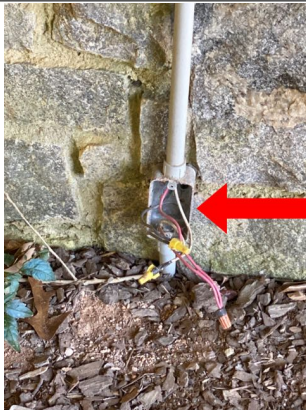
The conduit protecting the lower electrical wires on the rear side of the building was not safely installed. Recommend repair by qualified electrician.
