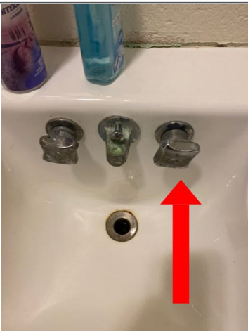
The sink cold water handle in the rear bathroom would not turn. Recommend repair by qualified plumber.
