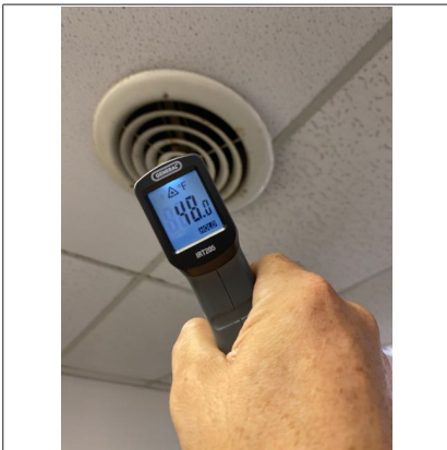
System two air conditioning temperature at register
