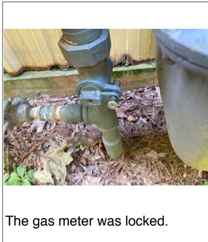
Main fuel shut off and gas meter located on right side of building
