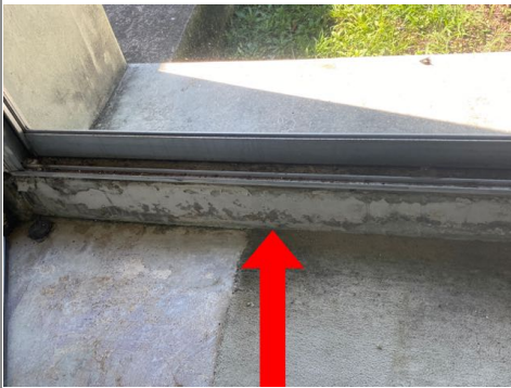
The moisture content was elevated in the walls below the windows in the police department. Recommend repair by qualified contractor.
