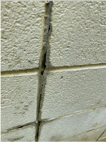
The block mortar needed to be re-pointed in several areas on the right side of the building. Recommend repair by qualified brick mason.
