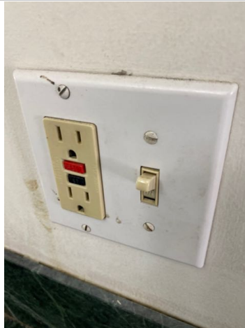
The GFCI electrical receptacle in the men's restroom was tripped and would not reset. Recommend repair by qualified electrician.
