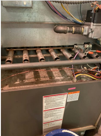
Furnace one would not ignite using the thermostat. Recommend repair by qualified HVAC technician.
