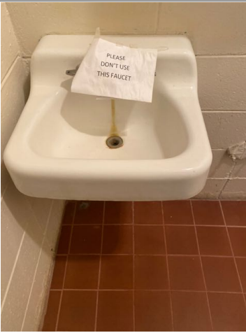
The sink in the bathroom in front of the registrars office was not working.
