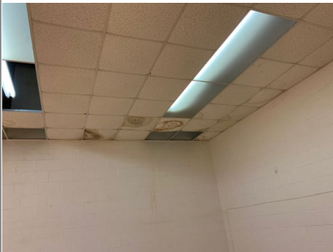
There were moisture stains on the ceiling in the rear right room but the moisture content was not elevated.
