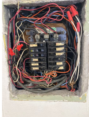
Interior of electrical sub panel three located in lower front side of building
