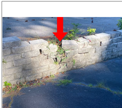
Several blocks were loose in the front left retaining wall. Recommend repair by qualified landscaper.
