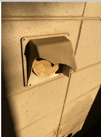
Recommend replacing the dryer vent cover located on the left side of the building.
