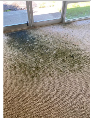
There was possible fungal growth on the flooring in front of the main entry doors. Recommend evaluation/repair by mold remediation specialist.
