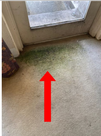
There was possible fungal growth on the floors in many areas in the sanctuary. Recommend evaluation/repair by mold remediation specialist.
