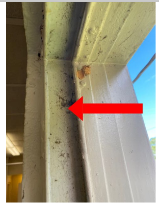
Recommend installing additional weatherstripping on the doors as needed.
