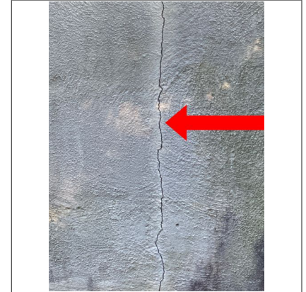
There were several cracks in the masonry veneer on the right side of the building that needed to be sealed.
