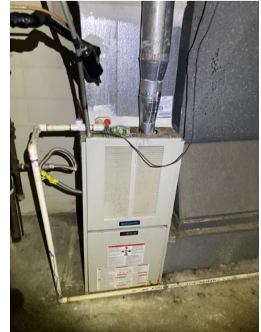
Interior HVAC system three located in front of bookstore
