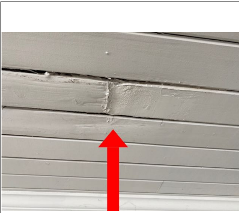
There was old moisture damage on the ceilings in several areas.
