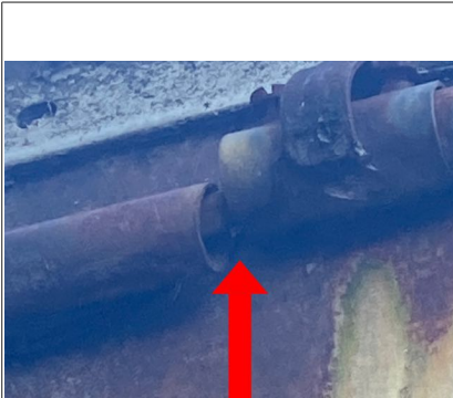
The conduit protecting the electrical wire to the light fixtures on the front side of the building was disconnected in several areas. Recommend repair by qualified electrician.
