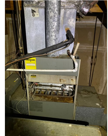
Interior HVAC system two located in attic
