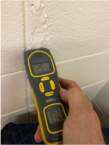
There were moisture stains on the front walls in several areas and the moisture content was elevated. Recommend repair by qualified contractor.
