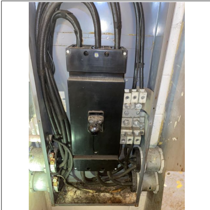
Interior of main electrical panel located in rear side of building
