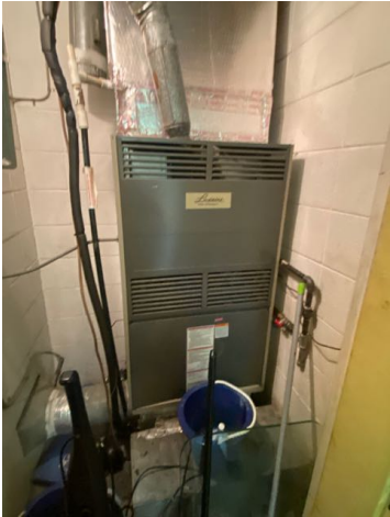
Interior HVAC system one located in front left utility closet
