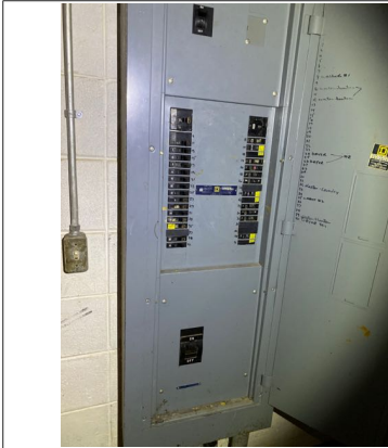
Main electrical panel located in laundry room
