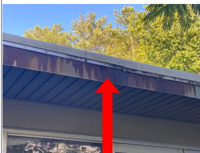
There was corrosion on the fascia on the right front side of the building. Recommend painting.
