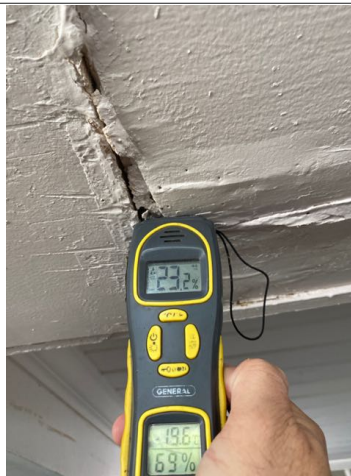
There was active moisture damage on the ceiling between the front entry and stairwell. Recommend repair by qualified contractor after the roof leaks are repaired.
