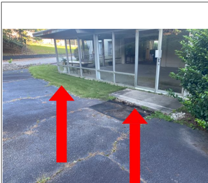
The grading was negative on the front side of the building and surface water appear to be entering through the entry doors. Recommend repair by qualified contractor.
