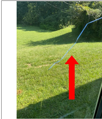
The glass was cracked in the left double door on the left side of the building. Recommend repair by qualified carpenter.
