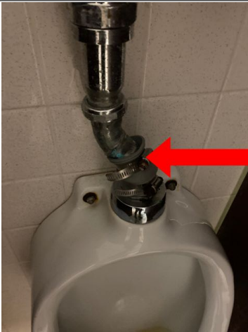
The plumbing had been poorly repaired on the right urinal in the men's bathroom. Recommend repair by qualified plumber.
