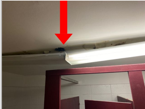
The ceiling light fixtures in the men's bathroom were not properly attached. Recommend repair by qualified electrician.
