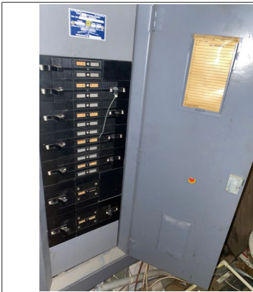
Recommend labeling all of the breakers in the electrical sub panel four.
