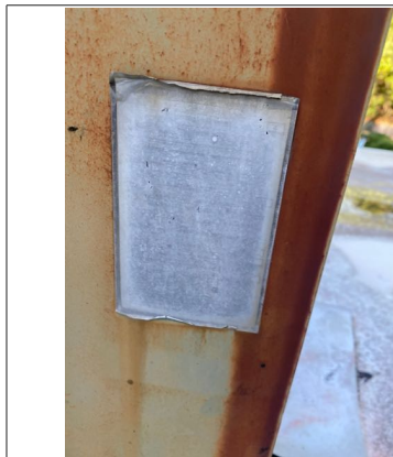
Unable to determine the exact age of exterior AC unit four because the manufacturer's data plate was not legible. It appeared to be 40+ years old.
