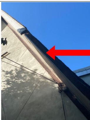
The fascia was missing on the rear left side of the building. Recommend repair by qualified carpenter.
