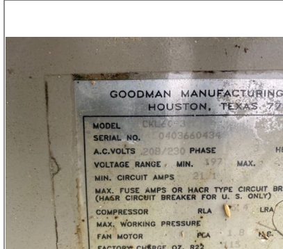
Exterior AC unit three
