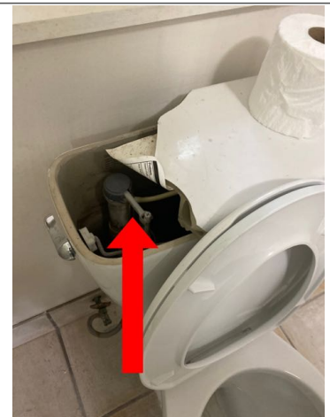
The left toilet lid tank in the women's bathroom was broken.
