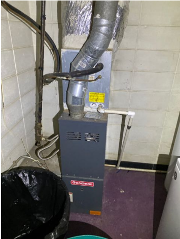
Interior HVAC system one located in laundry room
