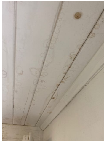
There was old moisture damage on the ceiling in the men's restroom in several areas.
