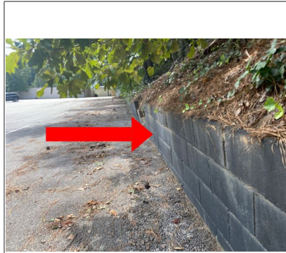
The block retaining wall on the right side of the main entrance was damaged in several areas and leaning. Recommend repair by qualified contractor.
