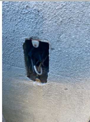
Recommended installing a cover plate on the electrical box on the left middle side of the building.
