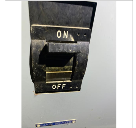
Main electrical disconnect two
