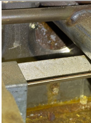
There was heavy corrosion inside furnace three. Recommend evaluation/repair by qualified HVAC technician.
