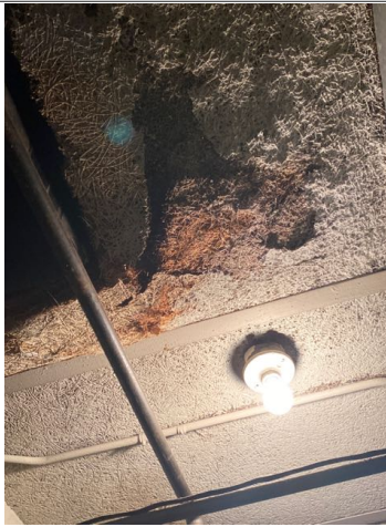
There was active moisture damage on the ceilings throughout the building. Recommend repair by qualified contractor.
