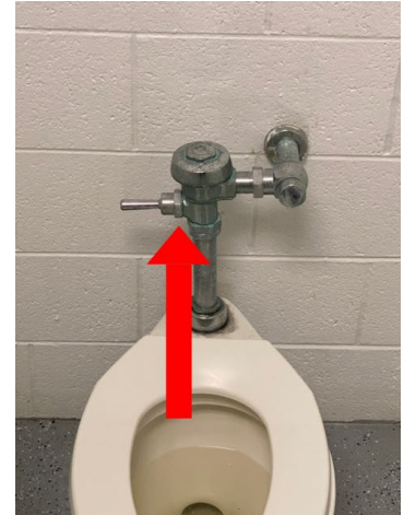
The left toilet in the rear left bathroom was leaking. Recommend repair by qualified plumber.
