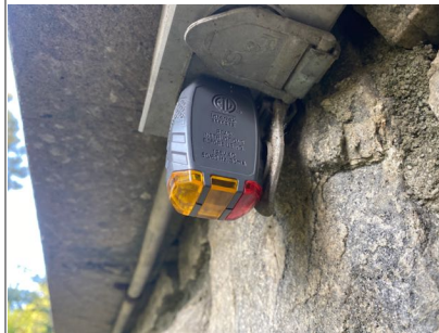
The electrical receptacle on the right side of the building was not working and did not appear to be GFCI protected. Recommend repair by qualified electrician.
