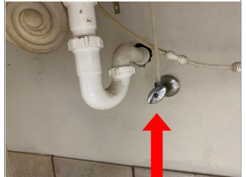
The water was turned off to the left sink in the women's restroom. It was not tested.
