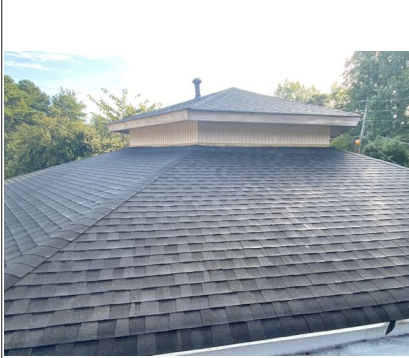
Overview of front slopes
