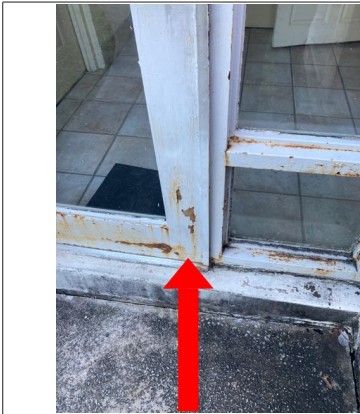
There was corrosion on the left entry doors and openings. Recommend painting.
