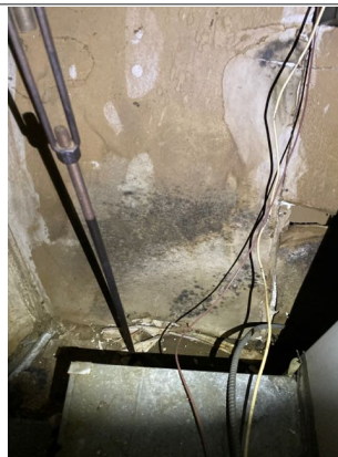
There was possible fungal growth on the attic walls. Recommend evaluation/repair by mold remediation specialist.
