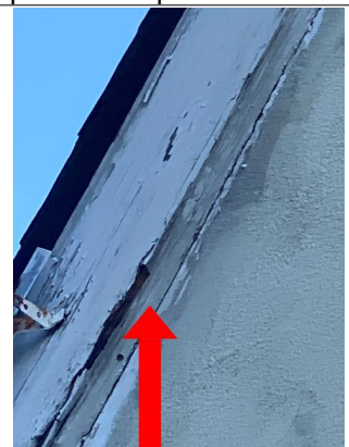
Recommend painting the wooden fascia on the front and rear sides of the building.
