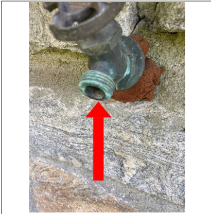
Recommend installing anti-siphon valves on the hose bibs.
