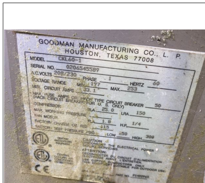
Exterior AC unit two
