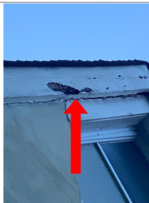
There was moisture damage on the upper fascia on the front side of the building. Recommend repair by qualified carpenter.
