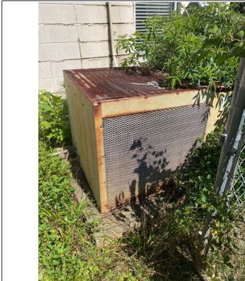
Exterior AC unit five located on left side of building
