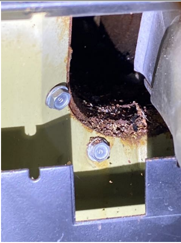
The interior of furnace four was heavily corroded. Recommend evaluation/repair by qualified HVAC technician.
