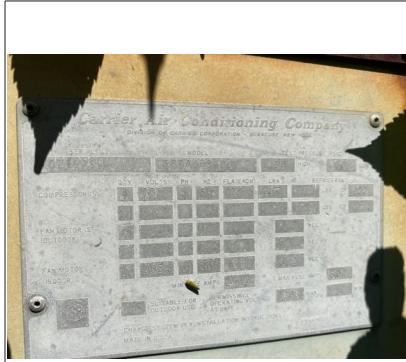
Unable to determine the exact age of exterior AC unit five. It appeared to be 45+ years old.
