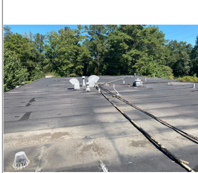
Front roof overview
