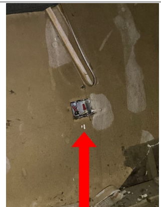
Recommend installing a cover plate on the electrical junction box on the front side of the attic.
