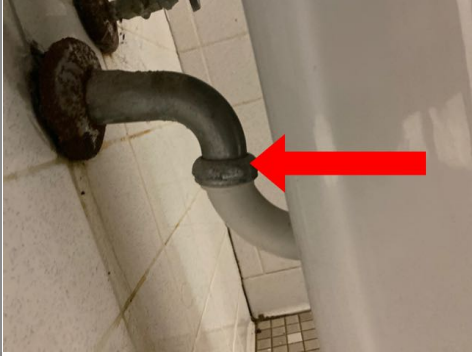
The right sink drain was leaking in the women's bathroom. Recommend repair by qualified plumber.
