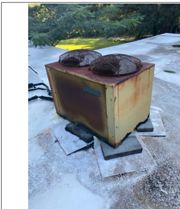
Exterior AC unit four was right unit located on front side of building
