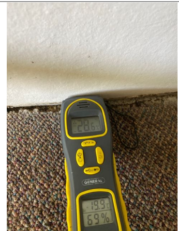
There was active moisture damage on the baseboards throughout the stairwell. Recommend repair by qualified contractor.
