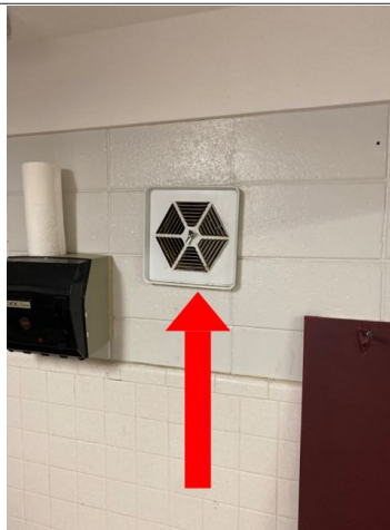
The ventilation fan in the women's bathroom was not working. Recommend repair by qualified electrician.
