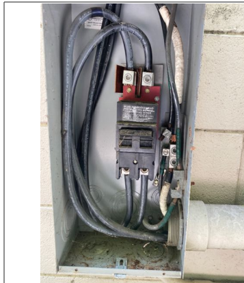
Interior of main electrical panel two located on right side of building
