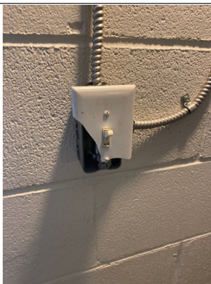
Recommend replacing the cover plate on the light switch on the rear left wall of the sanctuary.
