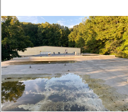
Rear roof overview
