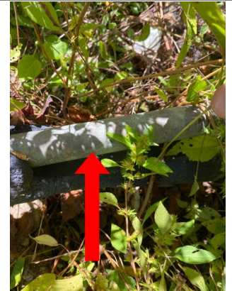
Recommend replacing the insulation on the suction line for exterior AC unit three.
