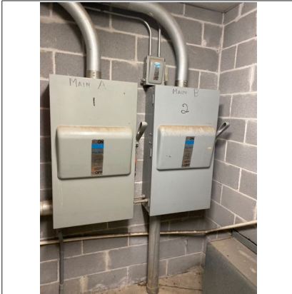
Main electrical disconnects located in left side of building
