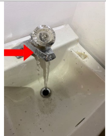
The sink faucet was leaking in the upper front right room. Recommend repair by qualified plumber.
