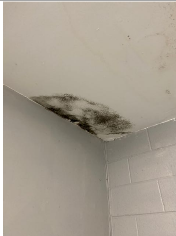
There was possible fungal growth on the ceiling in the front left room. Recommend evaluation/repair by mold remediation specialist.
