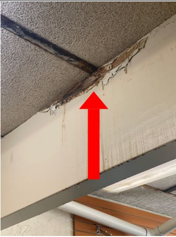
There was active moisture damage on the right beam in the bookstore. Recommend evaluation/repair by qualified contractor.
