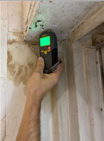
There was active moisture damage on the left side of the rear left entry doors. Recommend repair by qualified contractor.
