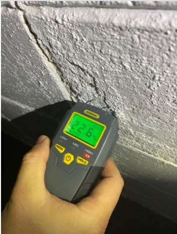
There was active moisture damage on the ceiling and walls in the front of the library. Recommend repair by qualified contractor after the roof is repaired.
