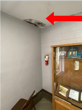
There was active moisture damage on the wall and ceiling in the front left room. Recommend repair by qualified contractor after the roof leak is repaired.
