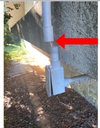
The conduit protecting the lower electrical wires on the rear side of the building was not safely installed. Recommend repair by qualified electrician.
