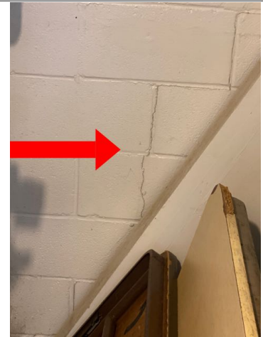
There was a minor vertical crack in the wall in the rear left side of the sanctuary. No action recommended.
