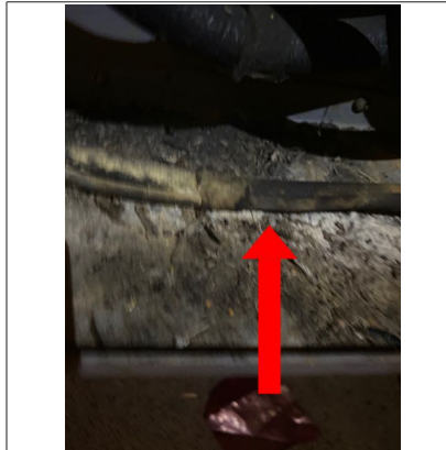
Wires in the bottom of the main electrical panel appeared to be scorched. Recommend evaluation by qualified electrician.
