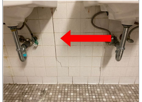
The wall tile was cracked underneath the sinks in the men's bathroom.
