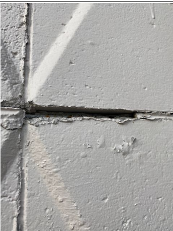
The block mortar needed to be re-pointed in several areas on the front side of the building. Recommend repair by qualified brick mason.
