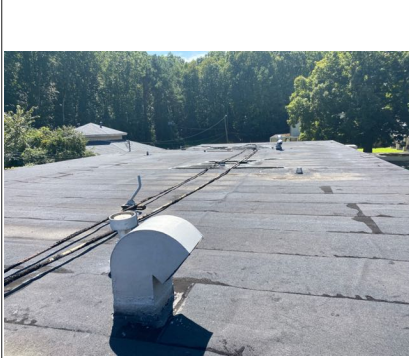
Rear roof overview
