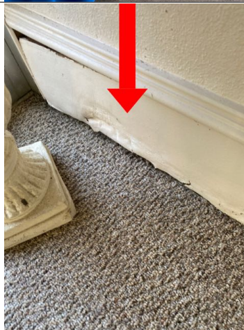
There was active moisture damage at the bottom of the rear walls in the front foyer. Recommend repair by qualified contractor.
