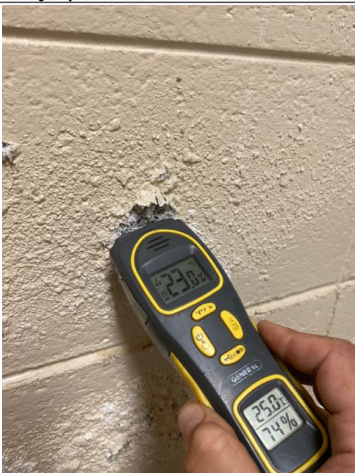
There were moisture stains on the left walls in several areas and the moisture content was elevated. Recommend repair by qualified contractor.
