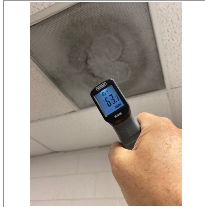
Several of the air conditioning systems were not cooling properly. Recommend repair by qualified HVAC technician.
