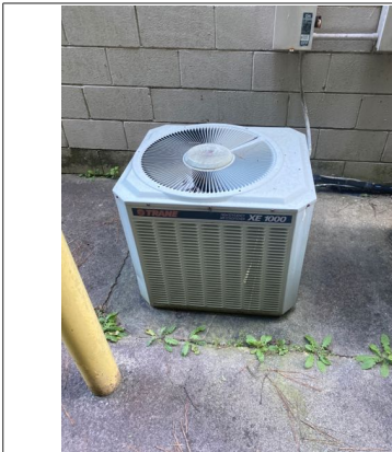
Exterior AC unit five located on right side of building
