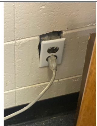
The electrical receptacle on the front wall of the conference room was not securely attached. Recommend repair by qualified electrician.
