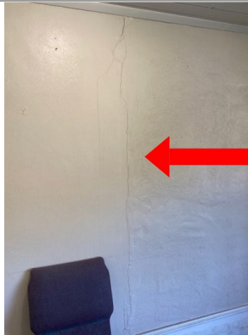
There was a crack in the front left wall of the sanctuary. No action recommended.
