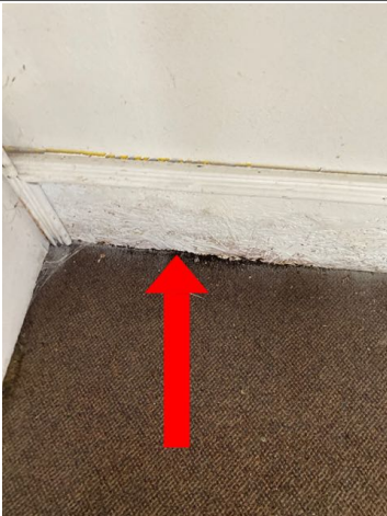
There was active moisture damage on the baseboards throughout the stairwell. Recommend repair by qualified contractor.
