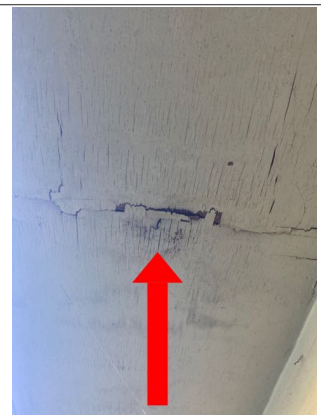
There was moisture damage on the soffit on the left front side of the building. Recommend repair by qualified carpenter.
