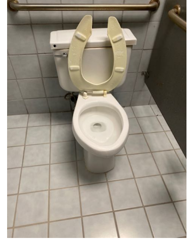
The left toilet in the rear boys bathroom was not securely attached to the floor. Recommend repair by qualified plumber.
