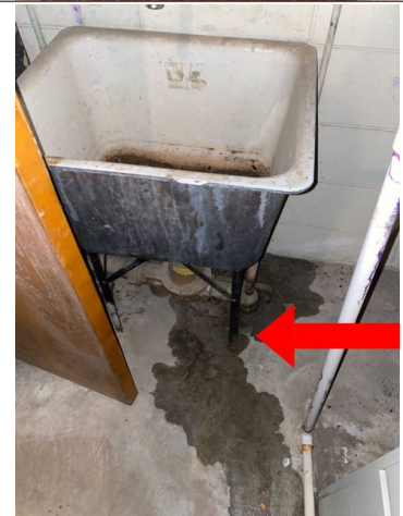
The drain for the utility sink in front of the bookstore was leaking. Recommend repair by qualified plumber.
