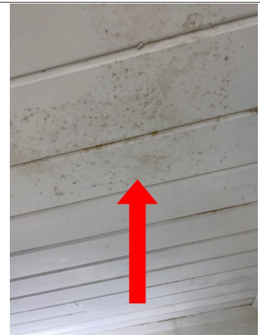
There was possible fungal growth on the ceiling in the men's restroom. Recommend evaluation/repair by mold remediation specialist.
