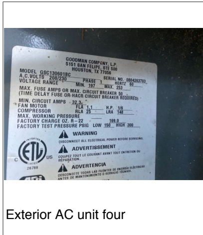
Exterior AC unit four located on right side of building
