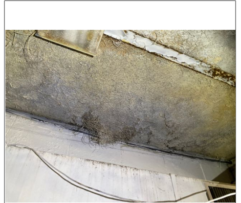
There was active moisture damage on the ceiling and walls in the front of the library. Recommend repair by qualified contractor after the roof is repaired.
