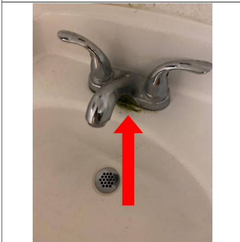
The left sink faucet in the men's bathroom was not securely attached. Recommend repair by qualified plumber.
