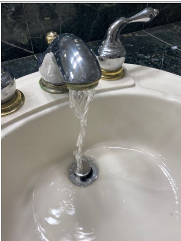
The hot water flow was poor in the women's restroom. Recommend repair by qualified plumber.
