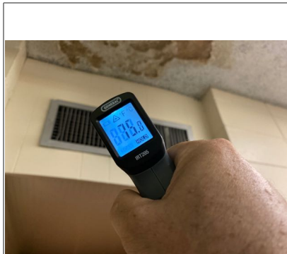
Air conditioning system two was not cooling properly. Recommend repair by qualified HVAC technician.
