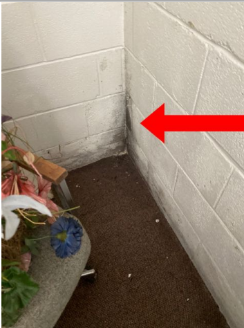
There was active moisture intrusion in the rear right corner of the building. Recommend repair by qualified contractor.
