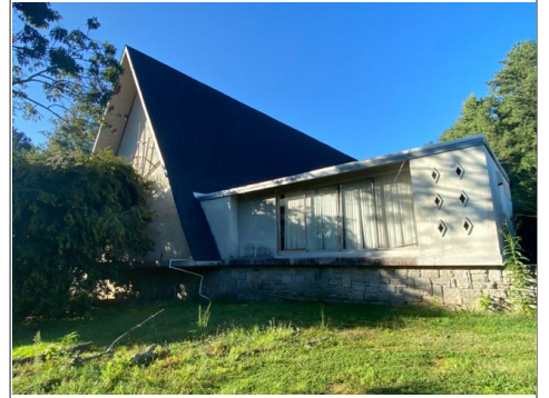
Rear elevation chapel
