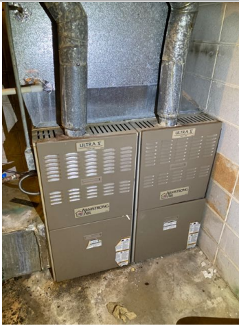
Interior HVAC system five located in rear side of building
