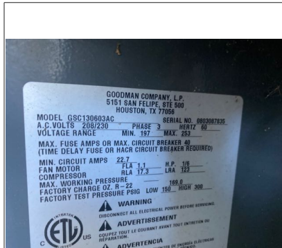
Exterior AC unit two
