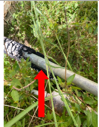
Recommend replacing the insulation on suction line for exterior AC unit five.
