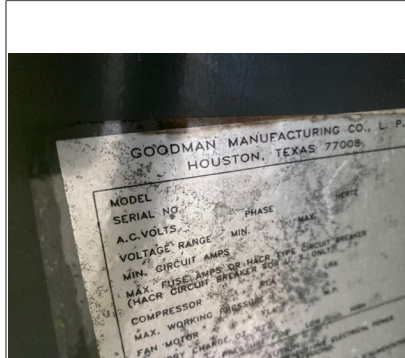
Unable to determine the exact age of exterior AC unit three because the manufacturer's data plate was faded. It appeared to be 12+ years old.
