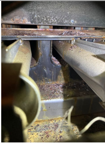
There was heavy corrosion inside furnace four. Recommend evaluation by qualified HVAC technician.
