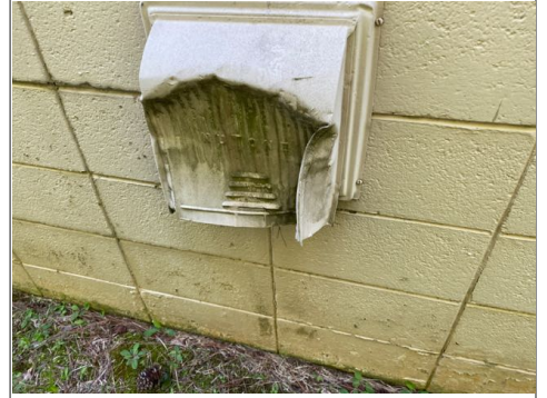
The vent cover on the right side of the building was damaged. Recommend replacement.
