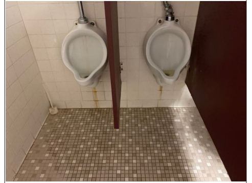
Both of the urinals in the men's bathroom were leaking. Recommend repair by qualified plumber.
