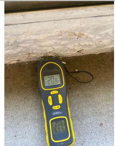
The moisture content was elevated in the walls below the windows in the chapel. Recommend repair by qualified contractor.
