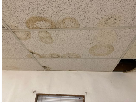
There was active moisture damage on the rear ceiling in the rear left room. Recommend repair by qualified contractor after the roof leaks are repaired.
