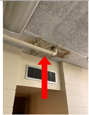
There was active moisture damage on the ceilings throughout the building. Recommend repair by qualified contractor.
