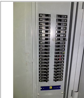
Electrical sub panel one located in right side of building
