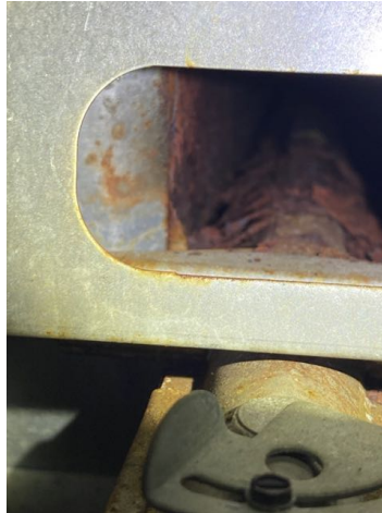
The interior of furnace two was heavily corroded. Recommend evaluation/repair by qualified HVAC technician.
