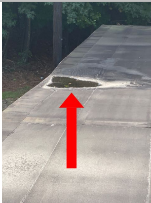
Water was ponding on the walkway covering on the left side of the gym where there was moisture damage on the ceiling of the walkway. Recommend repair by qualified roofer.
