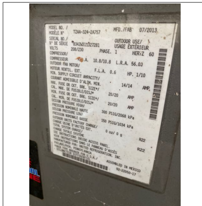
Exterior AC unit one
