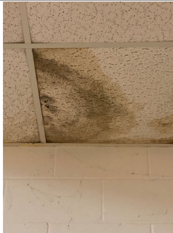
There was possible fungal growth on the ceiling tiles in the rear right room. Recommend evaluation/repair by mold remediation specialist.
