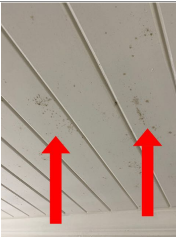
There was possible fungal growth on the ceiling in the women's bathroom. Recommend evaluation/repair by mold remediation specialist.
