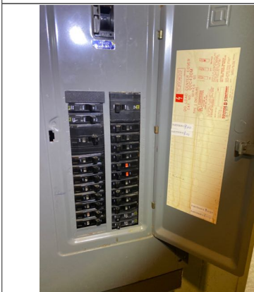
Recommend labeling all of the breakers in electrical panel three.
