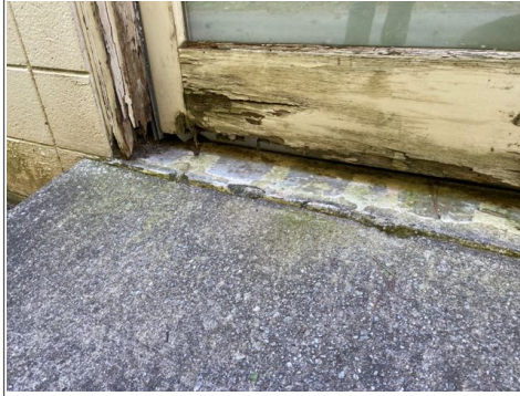
There was moisture damage on the door and door frame on the wooden door on the right side of the building. Recommend repair by qualified carpenter.
