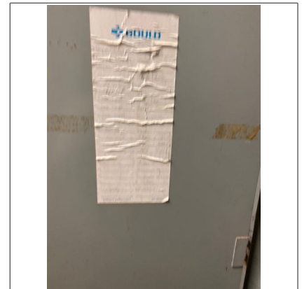
Recommend clearly labeling the breakers in electrical sub panel one.
