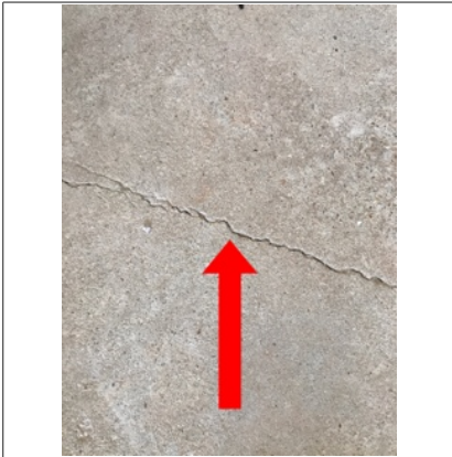
Typical cracks in garage floor. No action recommend.
