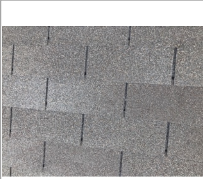
Overview of shingle condition
