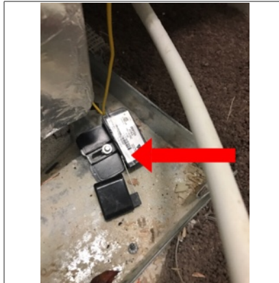
The overflow switch is disconnected from the pan on system one. Recommend repair by qualified HVAC technician.
