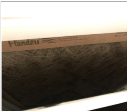
Recommend replacing the air filters.
