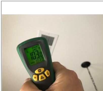
Heating system one temperature at register
